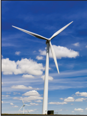
Pg. 5 - A large wind turbine provides off-grid power to build NH3 to be directly applied to the land.
