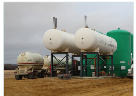
Pg. 12 - Farm storage at Hawk Hills, Alberta. Twin 30,000 gallon NH 3 tanks for 60,000 gallons Liquid App, ATS, KTS storage of 120,000 gallons is required.
